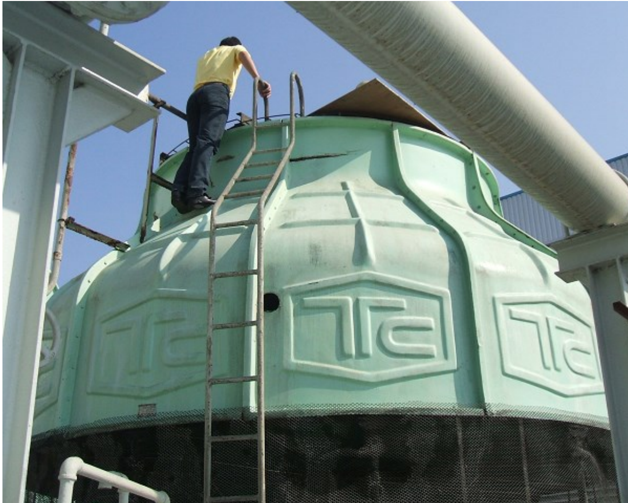
Aluminium Fans Removed
