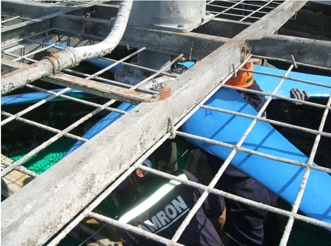
ENCON Blades Installed
