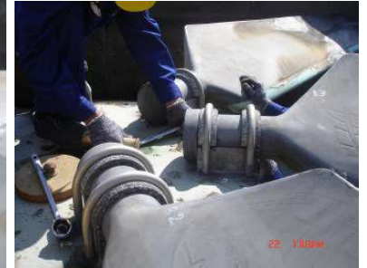
Existing Fans Removed (6 blades)
