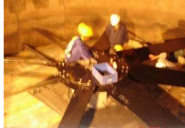
New ENCON Blades Installation & Angle adjustment
