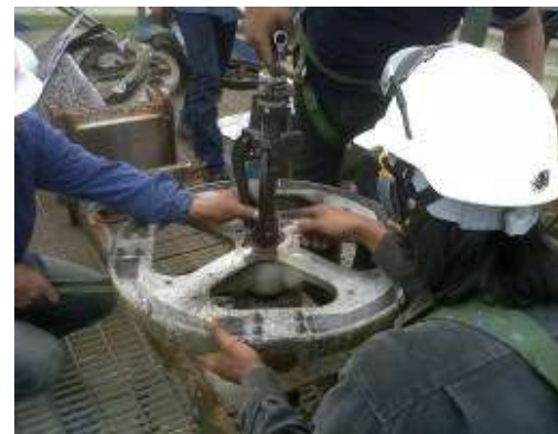
Existing Aluminium Fans & Hub Removed (4 blades)
